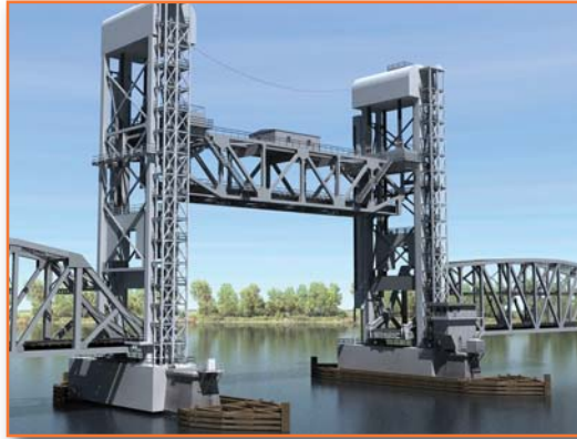
Pictured above is the newly refurbished Thames River Bridge located between New London and Groton, Connecticut .
